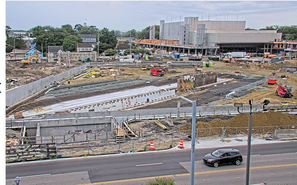
Atlantic Park Construction Progress as of 8/7/2024
