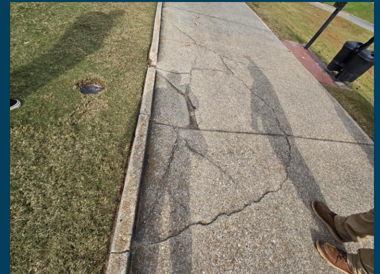
Drainage repair near hole 14
