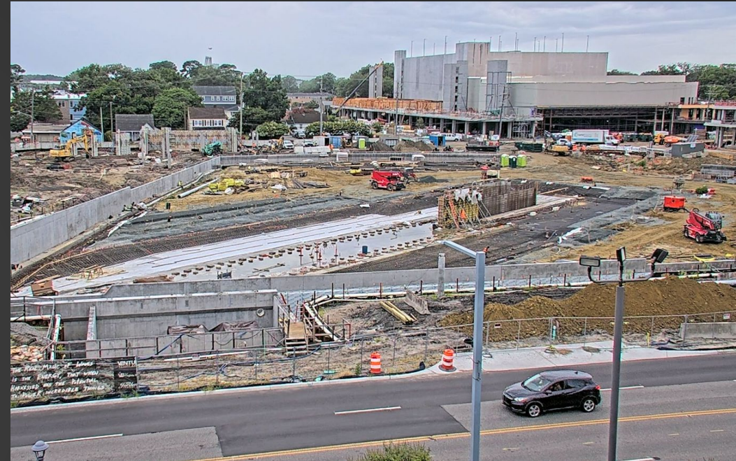
Atlantic Park Construction Progress as of 8/7/2024
